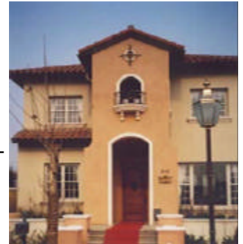
BMD supplied materials for the Napa Valley project near Beijing
