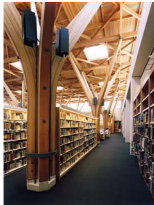
The delegation from Taiwan visited the Beaverton Library, a model of innovative design with glulams structural members.
