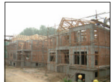
Wood frame hybrid construction at Vancouver Forest in Beijing.
